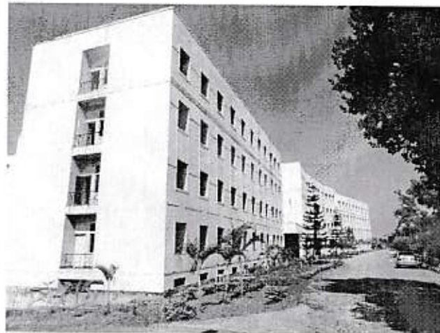
Front view of the Building
