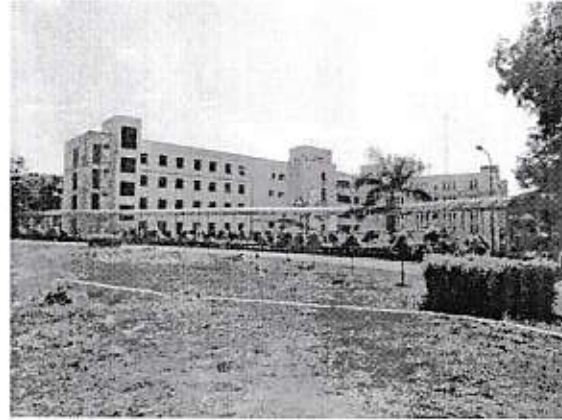
Rear view of the building
